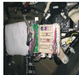
Rear Fuse Box
