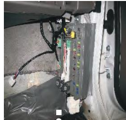
Pass. Under Dash Fuse/Relay Box
