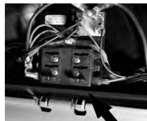
6-Way Fuse Box Behind Glove Box
