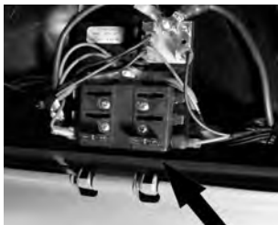
Remote Fuse Box Under Glove Box
