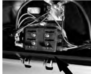
6-Way Fuse Box Behind Glove Box
